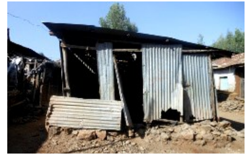
Toilet facilities before (above) and after (below) the project
